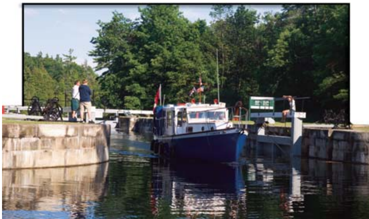
Davis Lockstation, Rideau Canal National Historic Site of Canada (ON), © Parks Canada, PHOTO: A. Guindon
